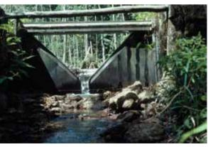
Photo 6.2. Weir to measure water flow, Kabo, 1982. (Photo K.E. Neering)
